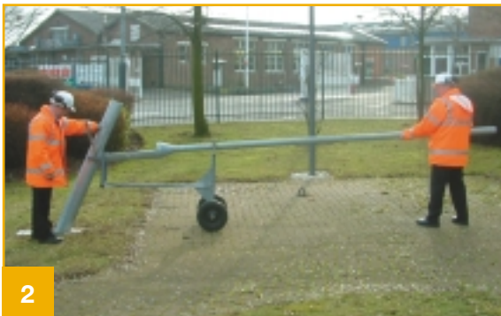
Lowering the root section into the foundation hole
