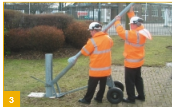
Raising the column to a vertical position
