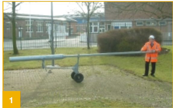
Column installed on the carrier and ready to install
