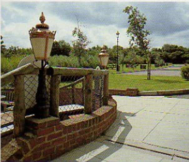
The Three Horseshoes Public House at Hooks Cross, Hertfordshire has a patio lit by Westminster Garden lanterns with opal glazing, on Lincoln pedestals.
