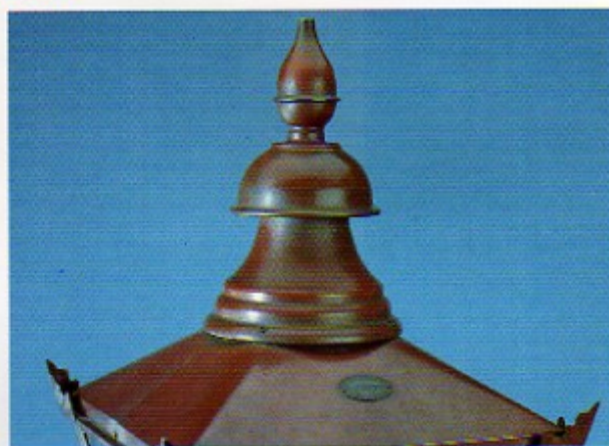
Detail of a weathered copper lantern.
