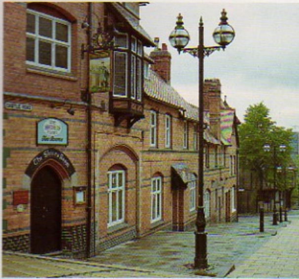
The Victorian architecture of this group of buildings in Castle Road, Nottingham, is emphasised by the double-arm mounted Richmond globes on Oxford lamp posts. Courtesy of Nottingham City Council.
