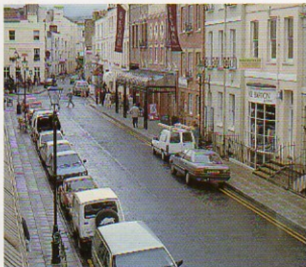
The elegance of Regent Street, Cheltenham, called for the installation of Windsor Street lanterns on Oxford lamp posts.
