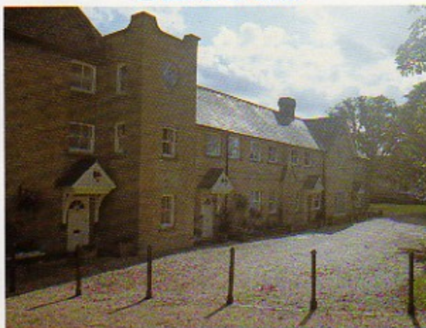
Hinged guard posts protect the tranquility of Courtyard Mews, Chapmore End in Hertfordshire.
