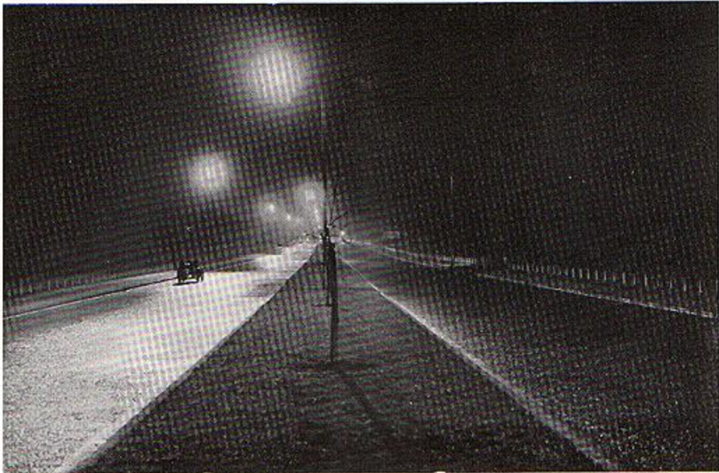
Both Carriageways are lighted with G.E.C. Uniway Lanterns and 125-Watt OSIRA Lamps. On each carriageway light is directed only towards on-coming traffic, making the other carriageway appear unlighted.
