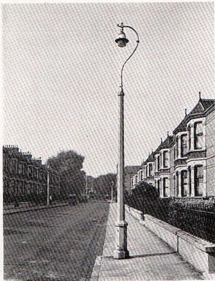
A concrete column for Side Street Lighting with small G.E.C. Lantern.
