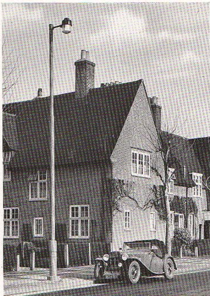
A modern steel Street Lighting Column, with G.E.C. Diffractor Lantern at 25-ft. mounting height.
