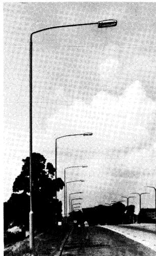
QA10 1090 on 8 m. steel column
