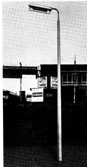
QB6 V/B2240.4 on steel column
