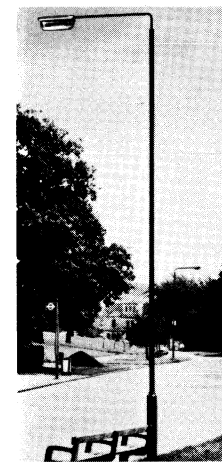
QA9 D 1090 on QLC M0887 column
