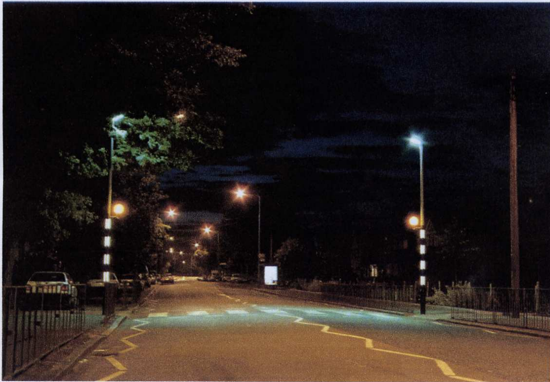
Night-time view showing the Zebrasafe Internally Illuminated Pole and the illumination of the crossing by overhead floodlight.
