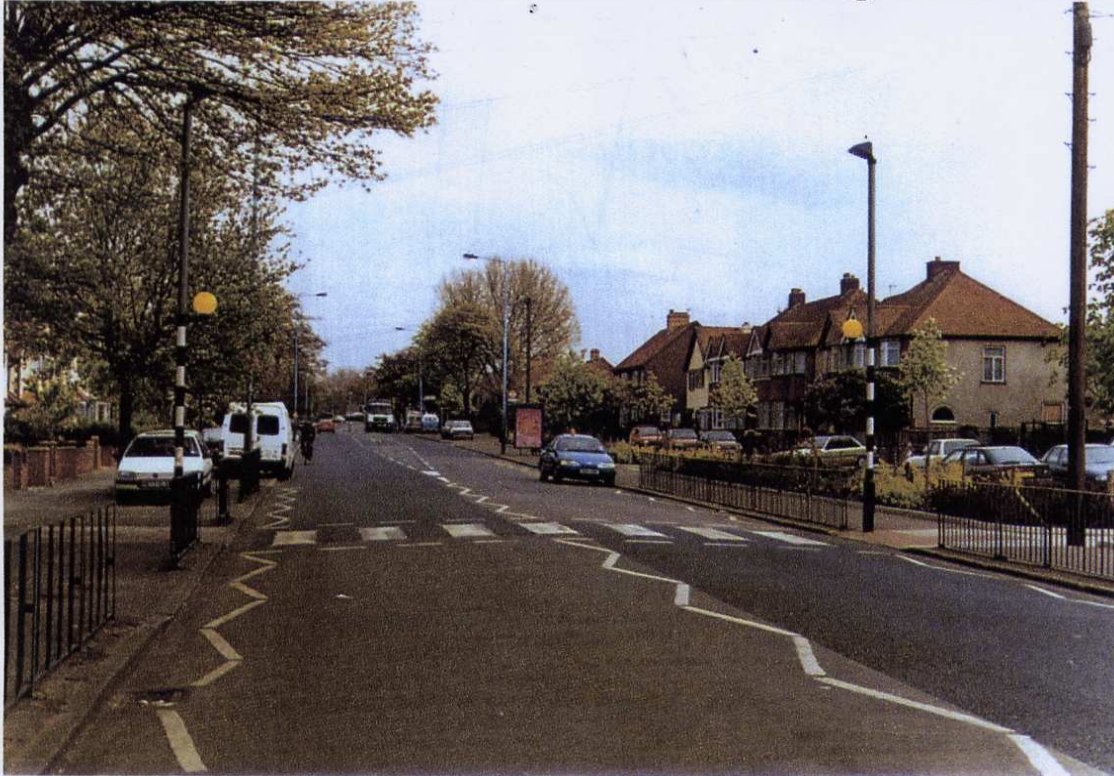
Daylight view of Installation.
