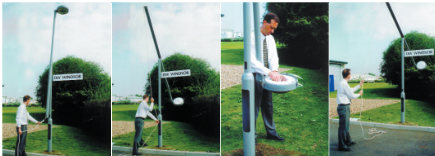
Lift the column away from the base
