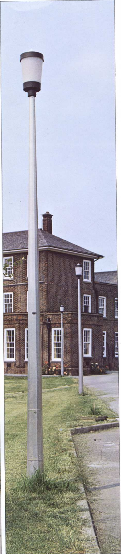
A Gamma 6 lantern on a Thorn aluminium column
