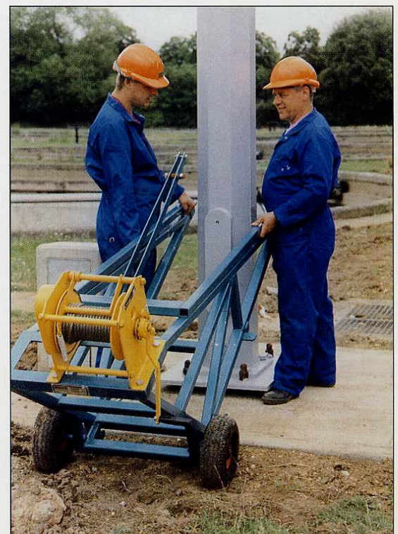
The Raising and Lowering Tool is offered up to the column
