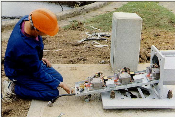
Control gear is accommodated in the base.
