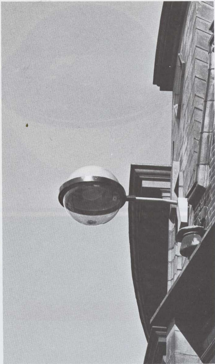
Photograph shows the P290 lantern at Norwich. Photograph by courtesy of D. Clark Esq., Dip., M.Illum.E.S., M.A.P.L.E., Lighting Engineer City of Norwich.
