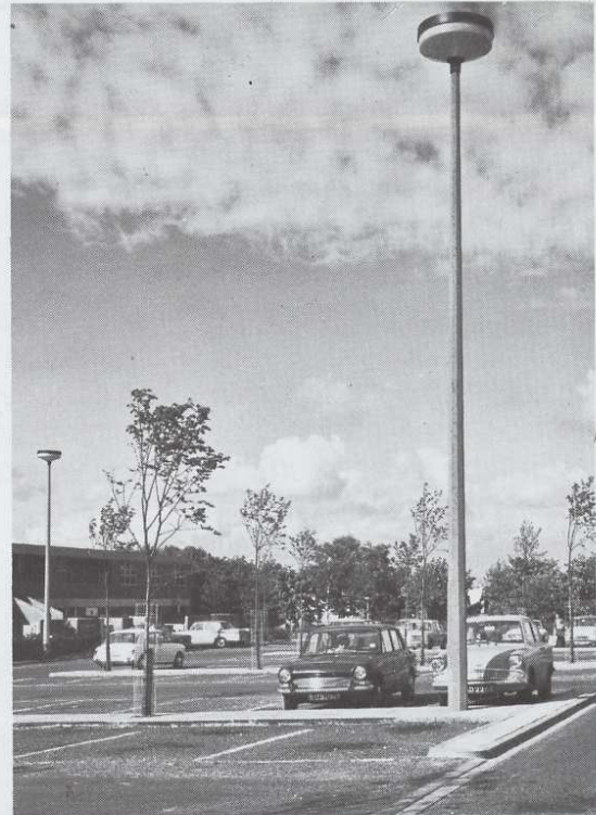
Photograph shows an installation of P222 lanterns on C.U. Limited's 'Highway' concrete columns, at Skelmersdale. Photograph by courtesy of D.H. Garside, CEng., FIMunE., MICE., AMInstHE., Chief Engineer, Skelmersdale Development Corporation.
