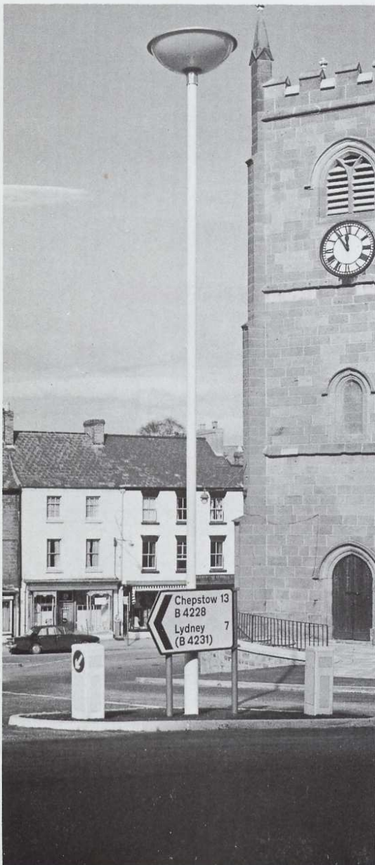
Photograph shows an installation of P.169 lanterns on steel columns at Coleford, Gloucester. Photograph by courtesy of West Dean R.D.C.
