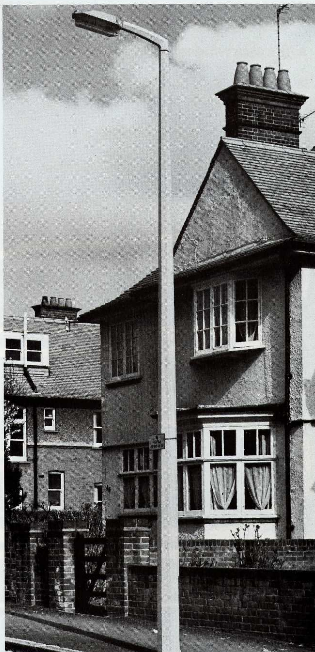
P226 lantern on a C.U. octagonal concrete column.
