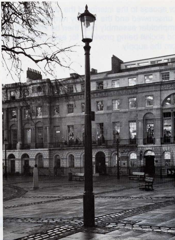
Phosco P109 lantern on a CU Fluted Column in Fitzroy Square, London. Photograph by courtesy of The London Borough of Camden.
