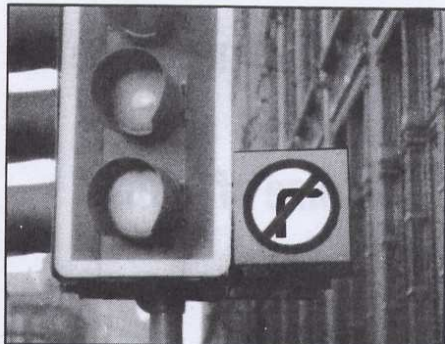
LIQUID CRYSTAL SIGN FITTED TO TRAFFIC SIGNAL
